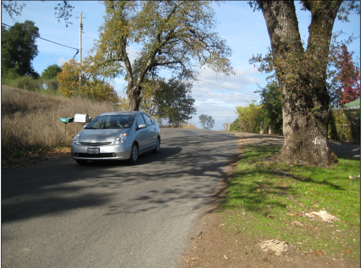
Photo 2: Looking on West Dry Creek Road towards the north from existing Seaton driveway (note limited visibility due to horizontal and vertical curves on roadway)
